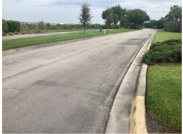
Ave Marie Blvd. – cracks and raveling evident
