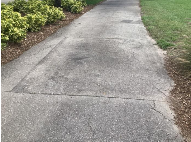
Cracks and previous repairs evident
