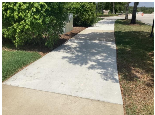
Concrete sidewalks – Anthem Parkway – partial replacements evident
