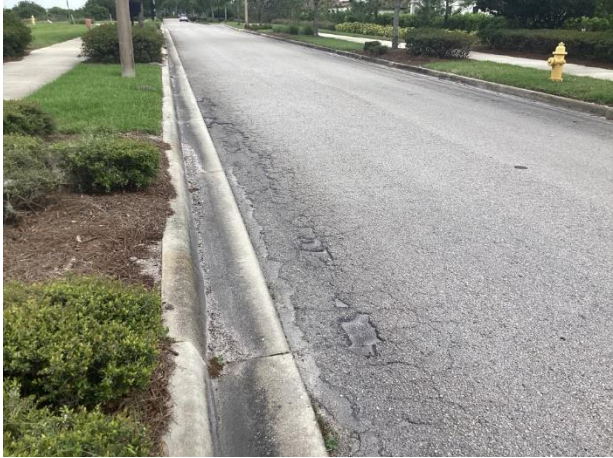
Pope John Paul Junior Blvd. – cracks and top layer deterioration evident
