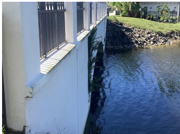
Vegetative growth evident – Seton St. bridge
