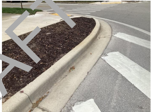
Concrete curbs and gutters - overview
