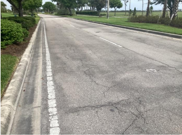
Ave Marie Blvd. – cracks and raveling evident
