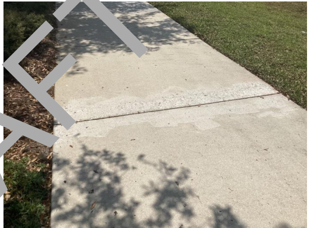
Concrete sidewalks – grinding repairs evident
