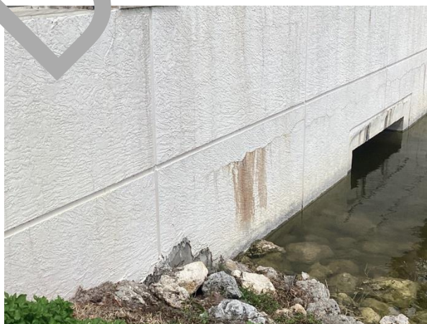
P Bridge – Pope John Paul II Blvd. – coating deterioration evident
