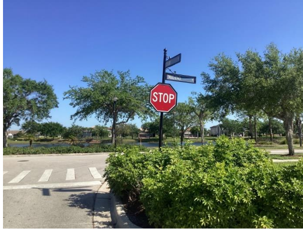
Signage – leaning sign posts evident
