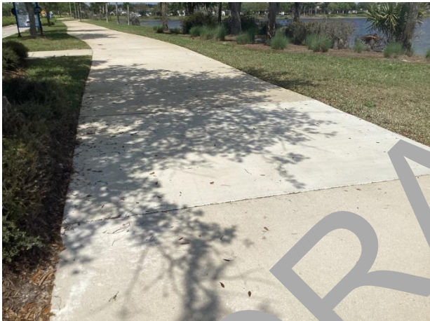
Concrete sidewalks – grinding repairs evident
