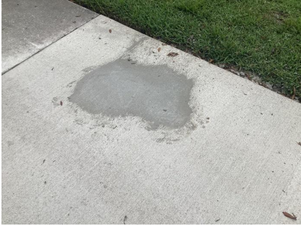
Concrete sidewalks – patch repairs evident
