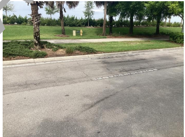
Ave Marie Blvd. – cracks and raveling evident
