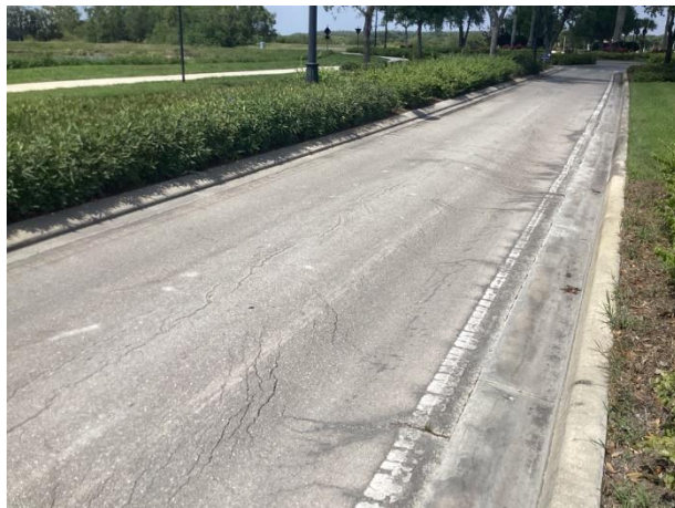
Ave Marie Blvd – cracks and raveling evident
