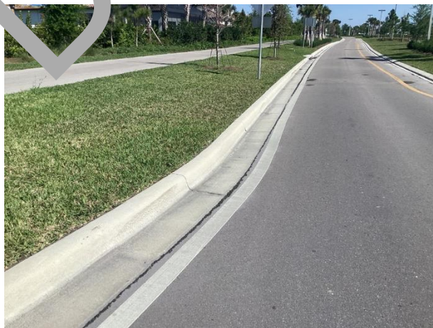
Concrete curbs and gutters - overview
