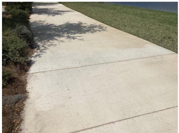
Concrete sidewalks – grinding repairs evident
