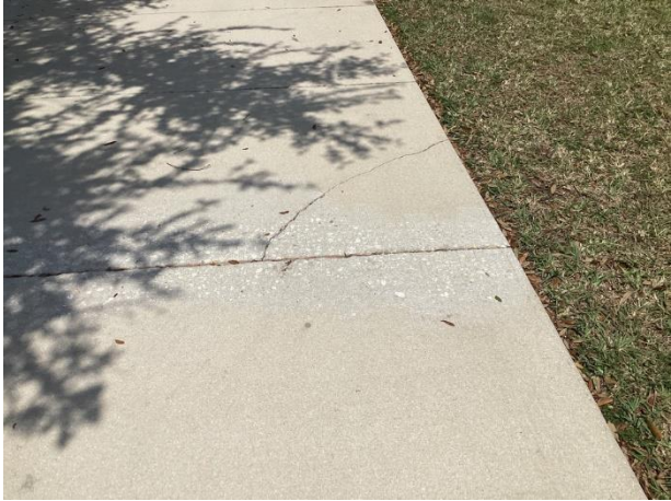
Concrete sidewalks – cracks and grinding repairs evident
