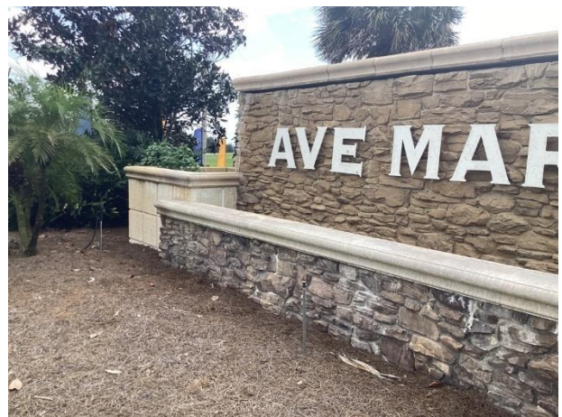
Stone veneer – minor efflorescence evident
