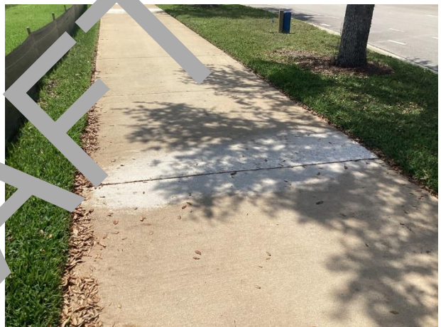
Concrete sidewalks – Anthem Parkway – grinding repairs evident
