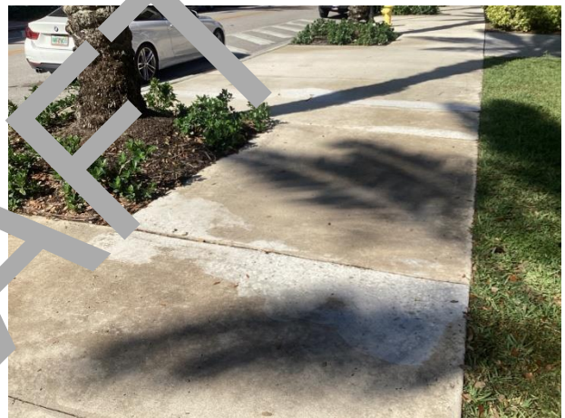
Concrete sidewalks – grinding repairs evident
