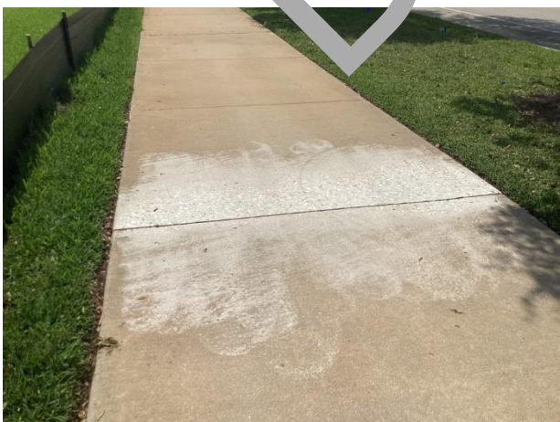
Concrete sidewalks – Anthem Parkway – grinding repairs evident
