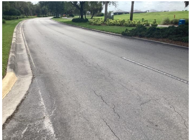
Ave Marie Blvd. – cracks and raveling evident
