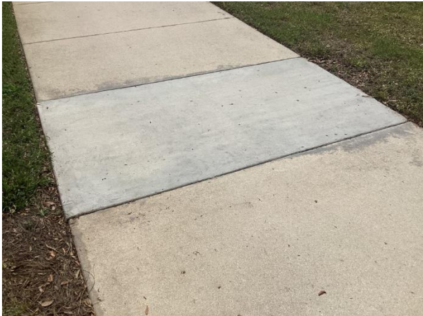
Concrete sidewalks – previous partial replacements evident
