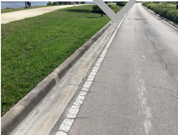
Concrete curbs and gutters - overview
