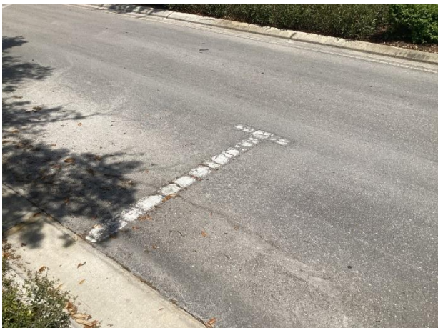
Ave Marie Blvd. – cracks and raveling evident
