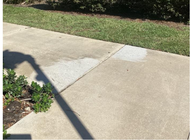
Concrete sidewalks – grinding repairs evident
