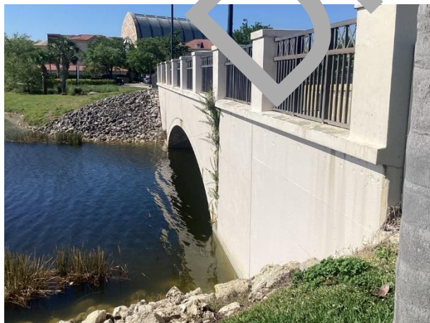
Vegetative growth evident – Seton St. bridge
