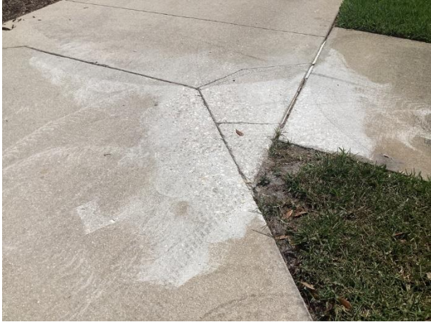
Concrete sidewalks - Ave Marie Blvd. – grinding repairs evident
