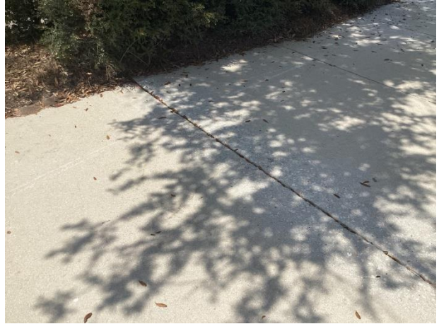
Concrete sidewalks – grinding repairs evident
