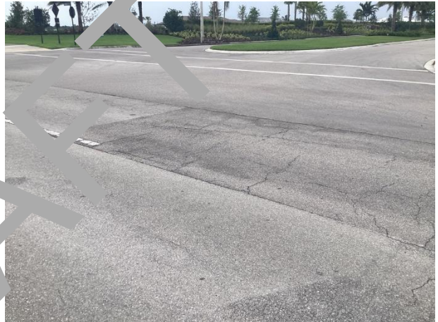
Ave Marie Blvd. – cracks and raveling evident
