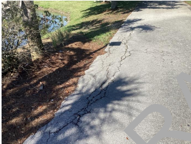
Asphalt pavement walking path - cracks evident
