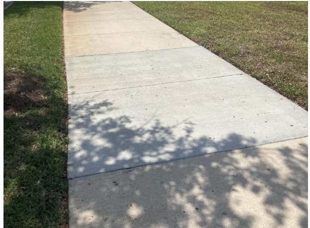
Concrete sidewalks – previous partial replacements evident
