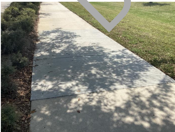
Concrete sidewalks – grinding repairs evident
