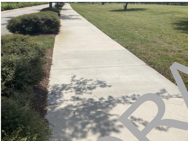
Concrete sidewalks – previous partial replacements evident
