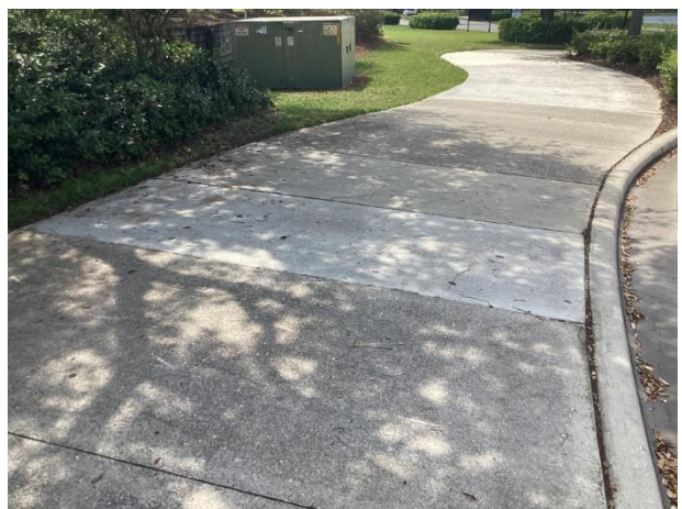
Concrete sidewalks - Ave Marie Blvd. – previous patch repairs evident
