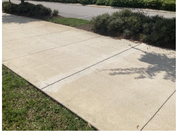
Concrete sidewalks - grinding repairs evident
