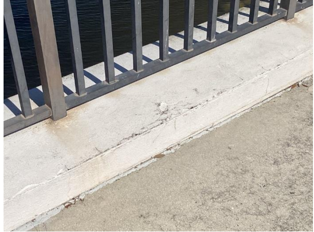
Bridges – coating fade evident
