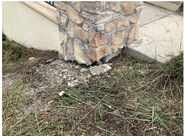
Bridge – Oil Well Rd. entrance – damaged masonry evident
