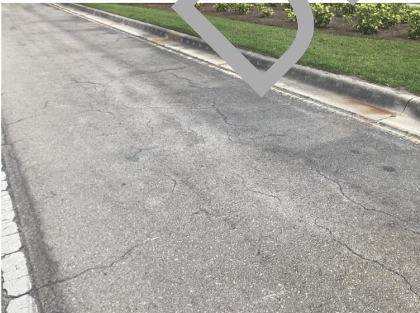
Ave Marie Blvd. – cracks and raveling evident
