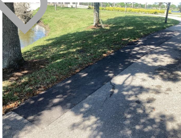
Asphalt pavement walking path – patch repairs evident
