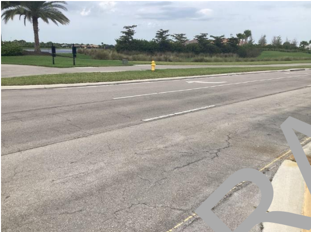
Ave Marie Blvd. – cracks and raveling evident
