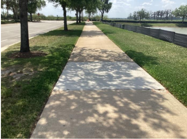
Concrete sidewalks – Anthem Parkway – partial replacements evident
