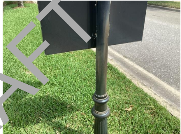
Signage – finish fade evident
