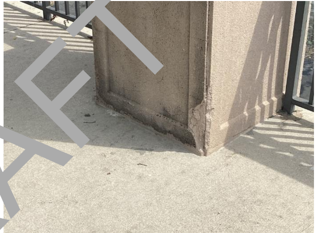
Bridge – Pope John Paul II Blvd. – coating deterioration evident
