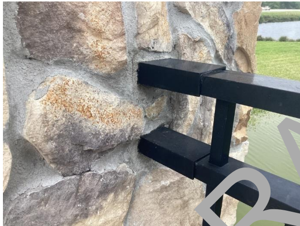
Railing connection - typical
