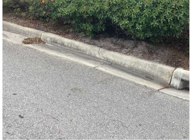
Concrete curbs and gutters – minor cracks evident
