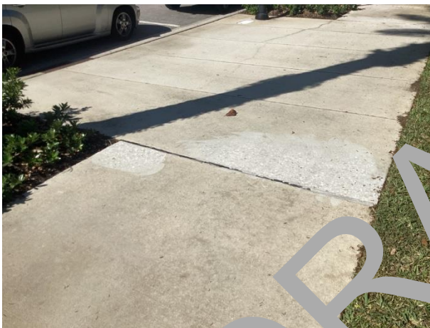
Concrete sidewalks – grinding repairs evident
