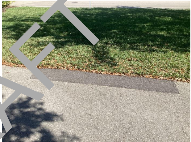
Asphalt pavement walking path – patch repairs evident
