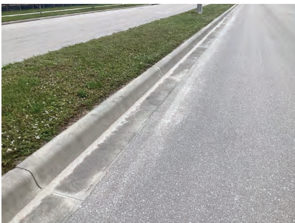
Concrete curbs and gutters - overview
