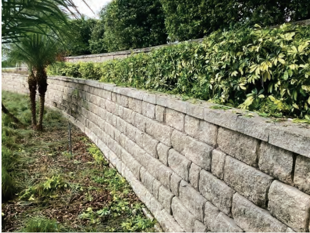
OWR retaining wall and landscaping
