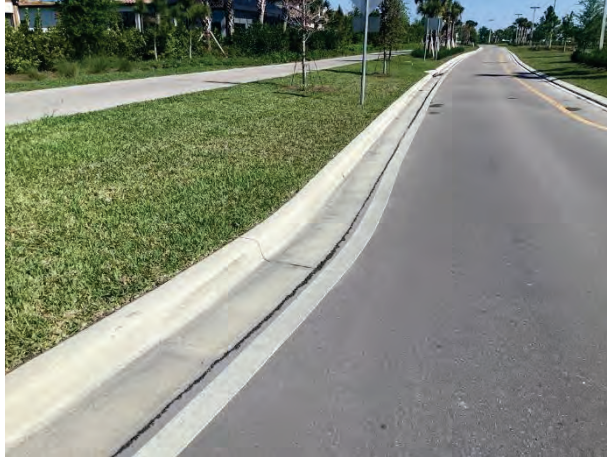
Concrete curbs and gutters - overview
