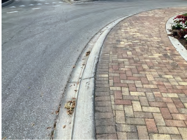
Concrete curbs and gutters - overview
