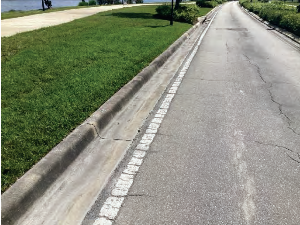
Concrete curbs and gutters - overview
