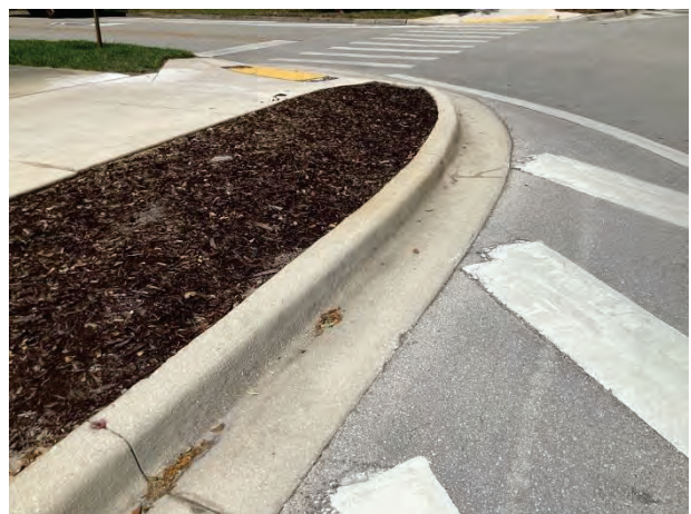
Concrete curbs and gutters - overview
