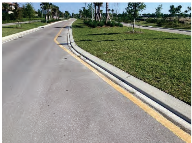
Concrete curbs and gutters - overview
