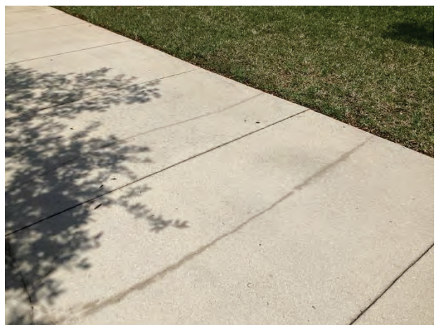
Concrete sidewalks - overview
