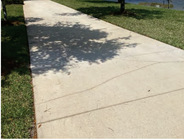
Concrete sidewalks - overview
