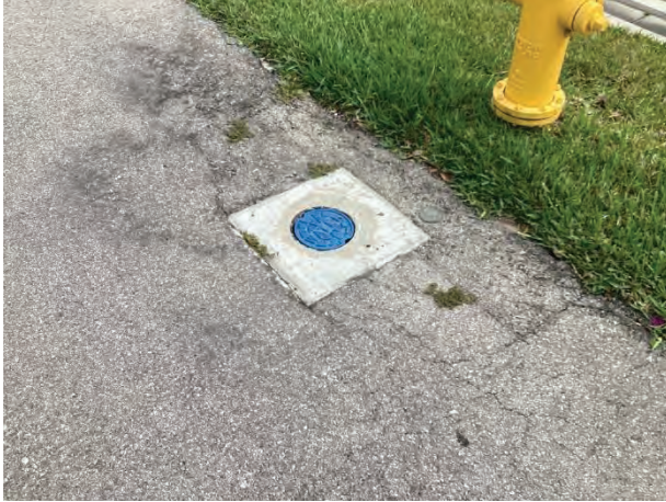
Cracks evident
