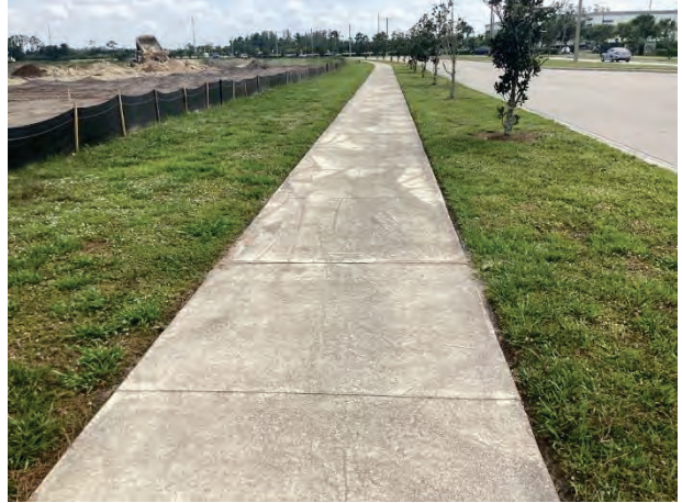
Concrete sidewalks - Arthrex Commerce - overview
