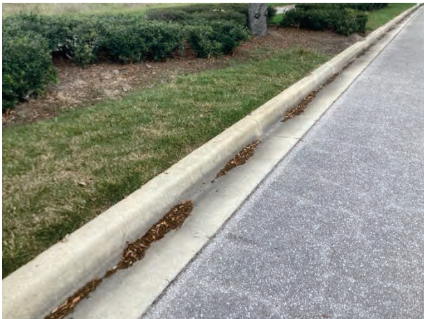
Concrete curbs and gutters - overview
