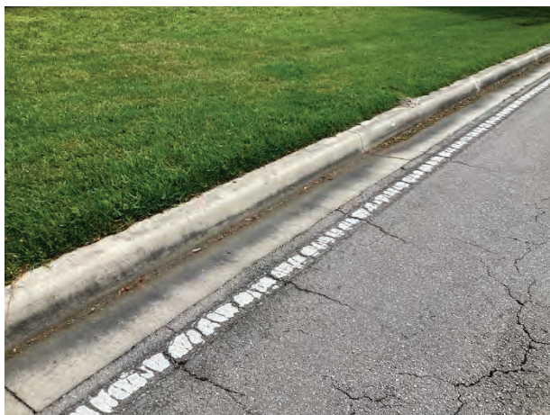
Concrete curbs and gutters - overview
