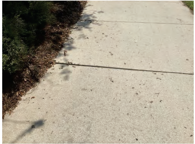
Concrete sidewalks – overview
