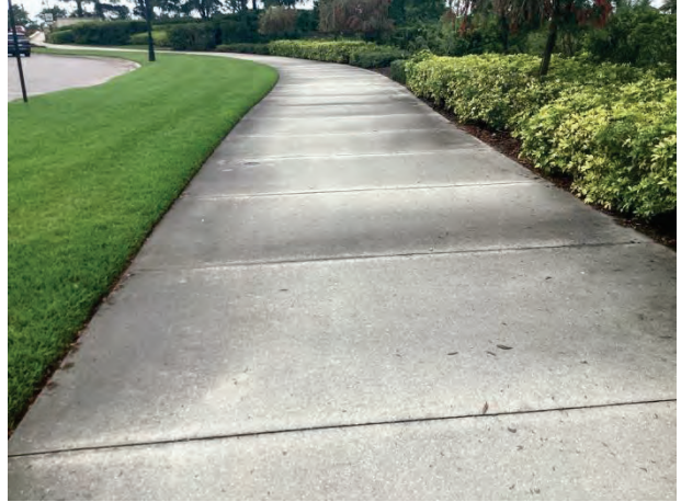
Concrete sidewalks - overview
