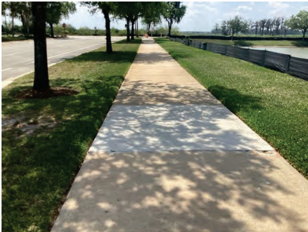
Concrete sidewalks – Anthem Parkway – partial replacements evident
