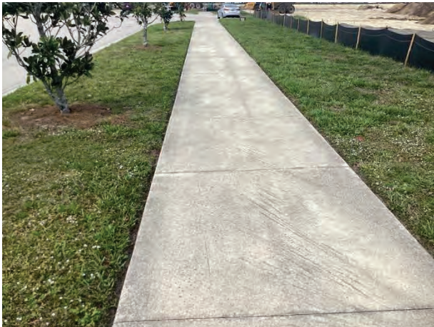
Concrete sidewalks - Arthrex Commerce - overview
