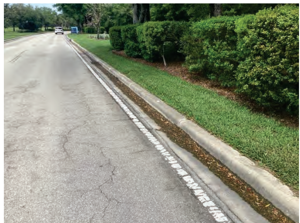
Concrete curbs and gutters - overview
