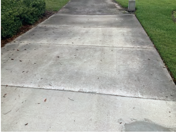
Concrete sidewalks - overview
