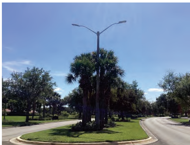
Light poles and fixtures – concrete - typical
