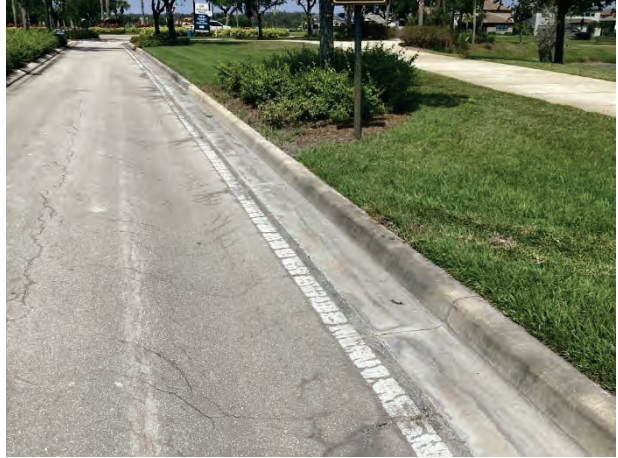
Concrete curbs and gutters - overview
