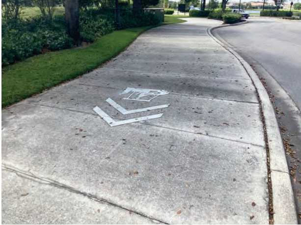
Concrete sidewalks - Ave Maria Blvd. – overview
