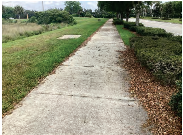
Concrete sidewalks – Pope John Paul II Blvd. - overview
