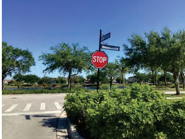
Signage – leaning sign posts evident
