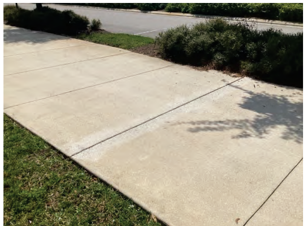
Concrete sidewalks - gridding repairs evident
