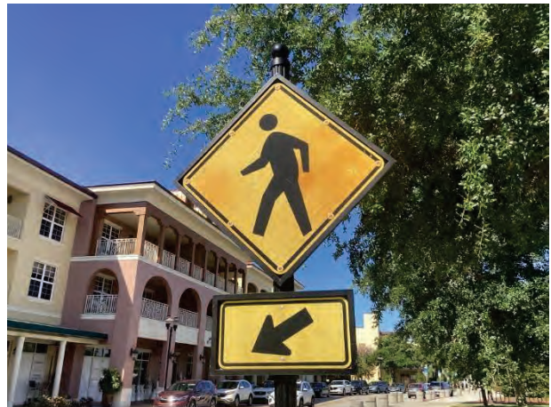
Signage – sign deterioration evident
