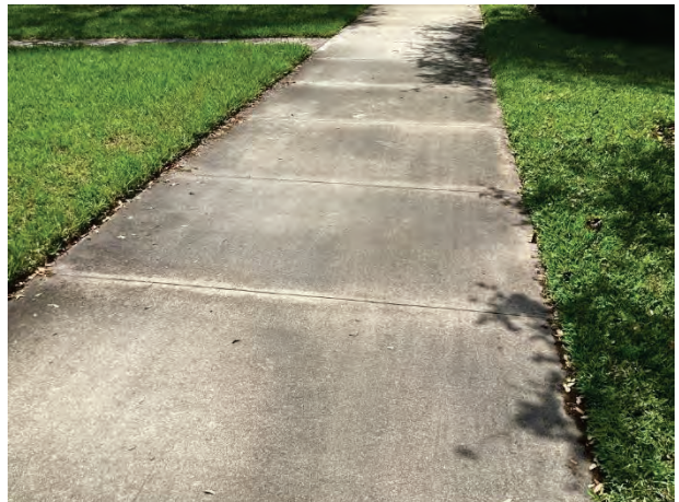
Concrete sidewalks - overview
