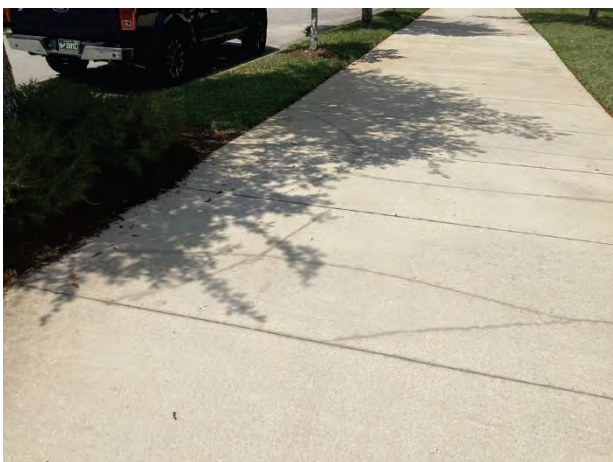
Concrete sidewalks - overview
