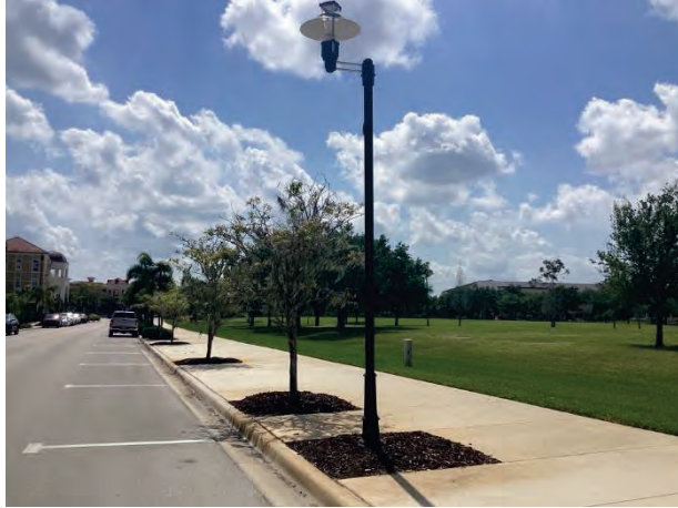
Light poles and fixtures – fiber glass - overview
