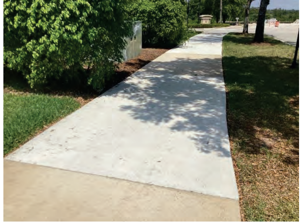
Concrete sidewalks – Anthem Parkway – partial replacements evident
