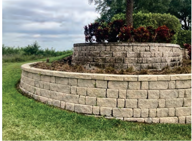
OWR retaining wall and landscaping
