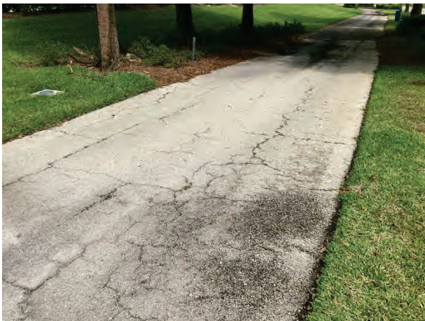
Cracks evident
