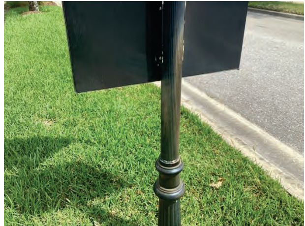
Signage – finish fade evident
