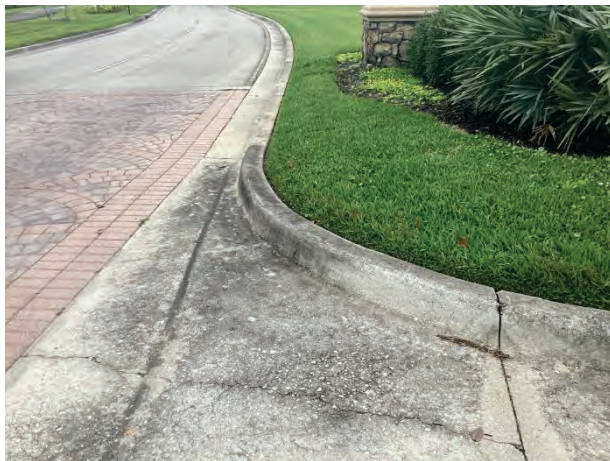
Concrete curbs and gutters - overview
