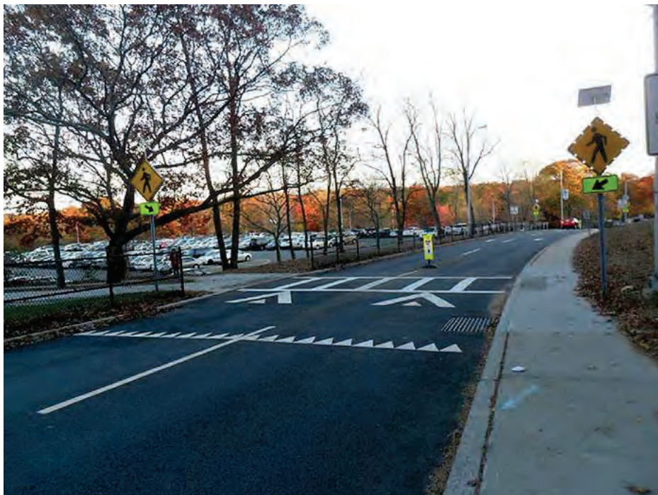
Figure 3.14.3. Raised Crosswalk Midblock (Source: R. Goldberg)
