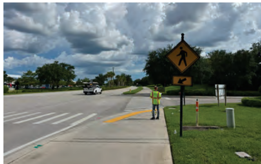
Figure 8: Southbound Pedestrian Warning Sign (W11-2) with Arrow Plaque (W16-7P) and Northwest Curb Ramp
