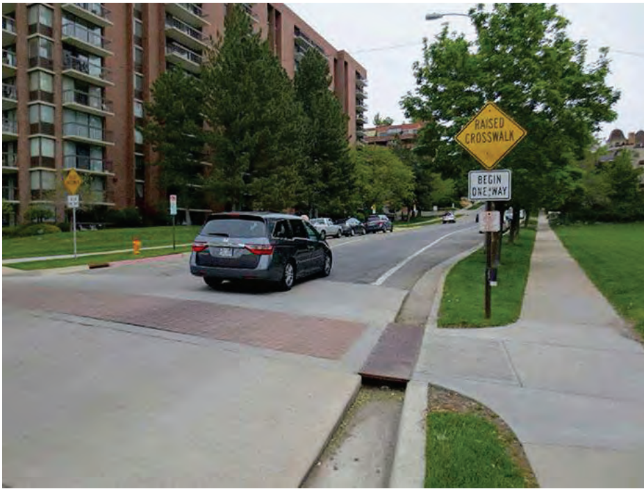
Figure 3.14.7. Raised Crosswalk Design to Accommodate Drainage (Source: Jeff Gulden)
