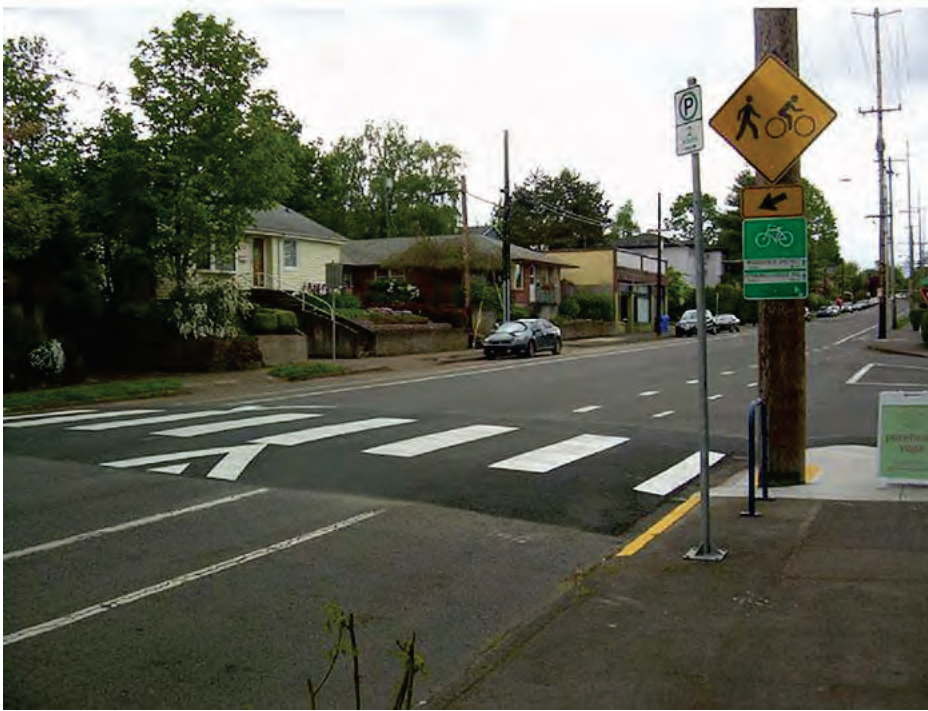
Figure 3.14.6. Raised Crosswalk with Bicycle Lane
