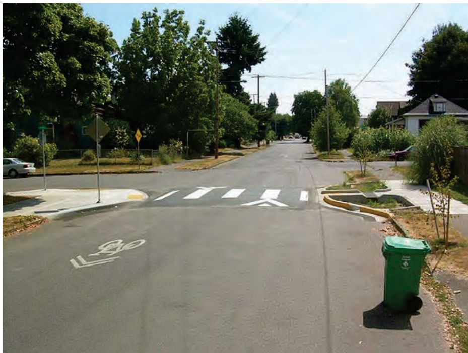
Figure 3.14.5. Raised Crosswalk with Curb Extension (Source: Scott Batson)
