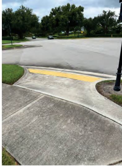
Figure 4: Curb Cut with Detectable Warning Mat, NE Corner
