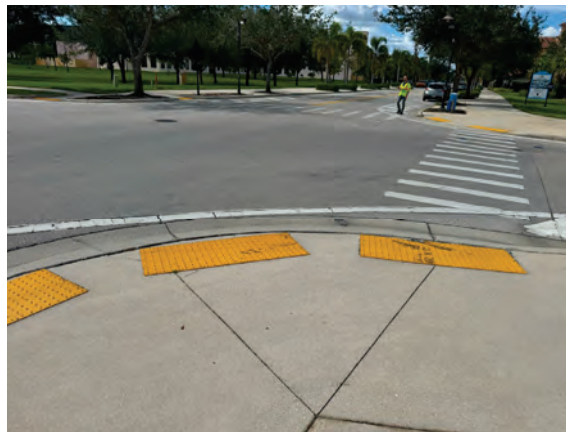
Figure 12: Southeast Corner Detectable Warning Mats
