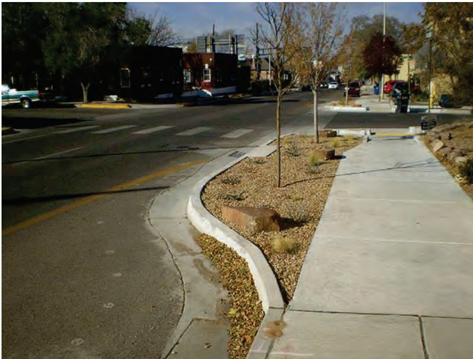
Figure 3.16.8. Corner Extension with Drainage Structure Relocation (Source: James R. Barrera)
