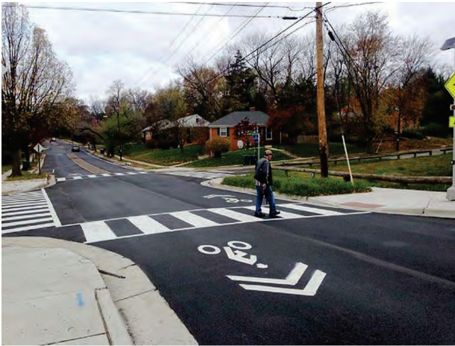
Figure 3.16.2. Corner Extension with Shortened Pedestrian Crossing Distance (Source: Hillary Orr)
